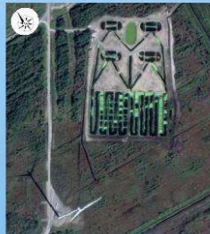
Figure 1: Aerial view of the AquaMona trial fish farm located in the middle of Mount Lucas Wind Farm, Co. Offaly. The wind turbine used to provide all electrical requirements is displayed in the bottom left-hand side of the image.
