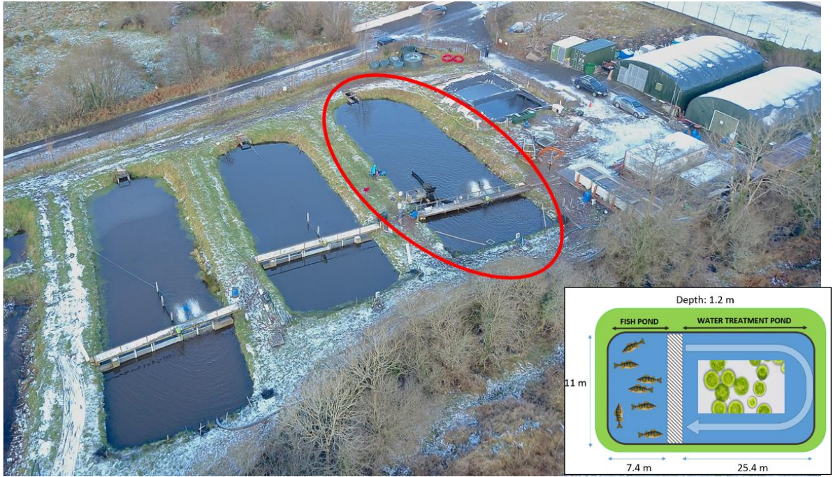
138 139 Fig. 1. Perch farm flow through ponds - aerial view, with insert schematic of Pond 1 layout.
