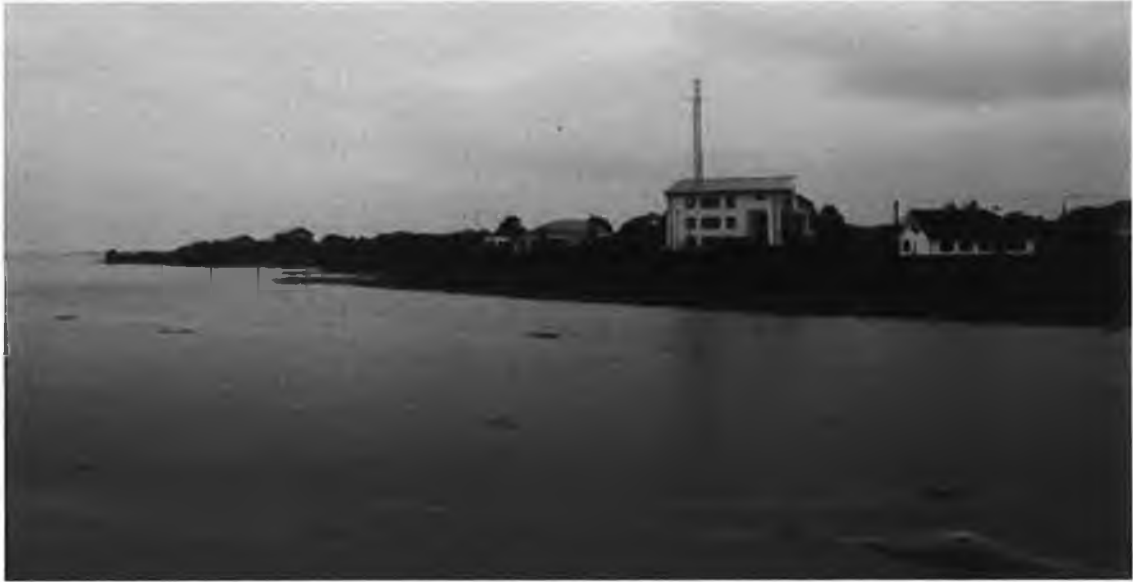
Figure 17: Pumping station and Garda station, Oranmore to the right of Photograph
