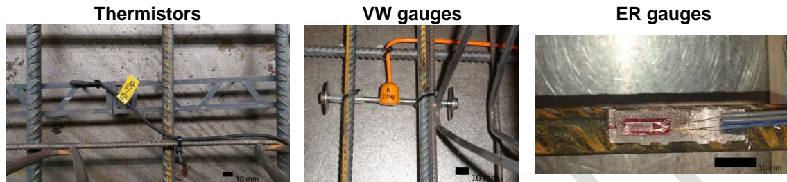
Figure 3. Sensors embedded in the building's structure
