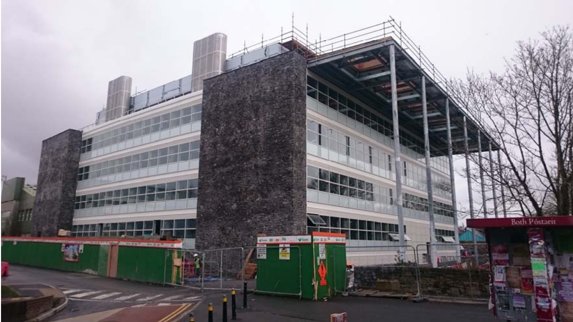
Figure 1. Human Biology Building (under construction)
