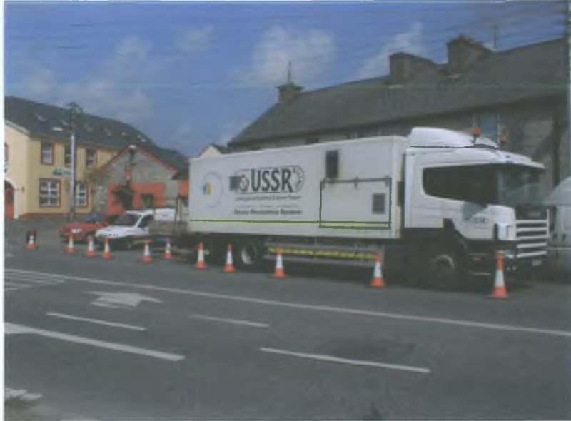
Photo 1. Typical rehabilitation truck working over manhole.
