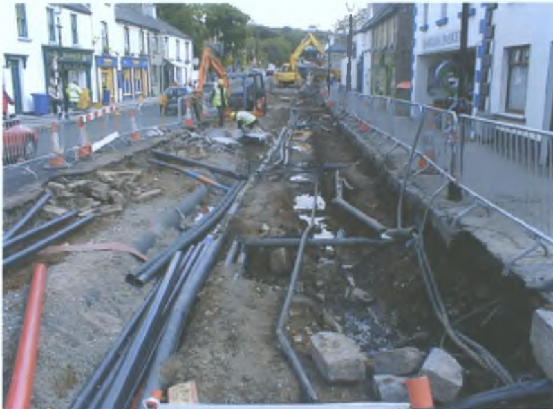
Photo 2. Typical open cut trench.
