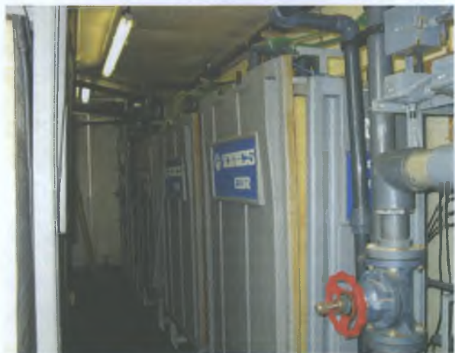
Plate 3: Membrane Stacks in series
