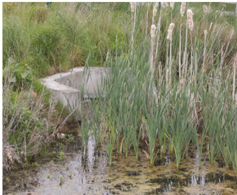
Photo 4.5 Settlement Pond Outlet
