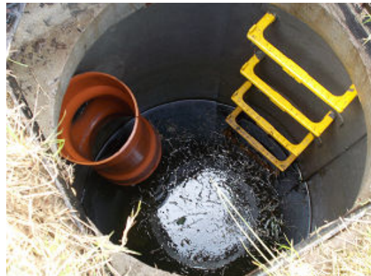
Photo 4.6: Interceptor Chamber
