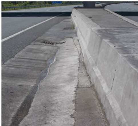
Photo 4.3: Gully Drain
