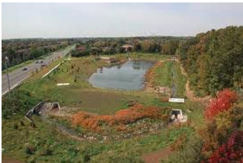
Photo 5.1: Stormwater Settlement Pond ( www.planningontario.com ) No scale specified
