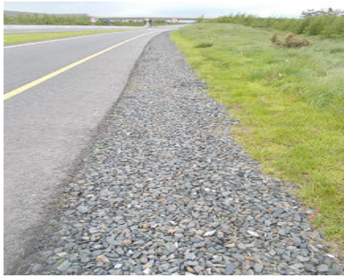
Photo 4.1: French Drain
