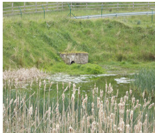
Photo 4.4: Inlet to Settlement Pond
